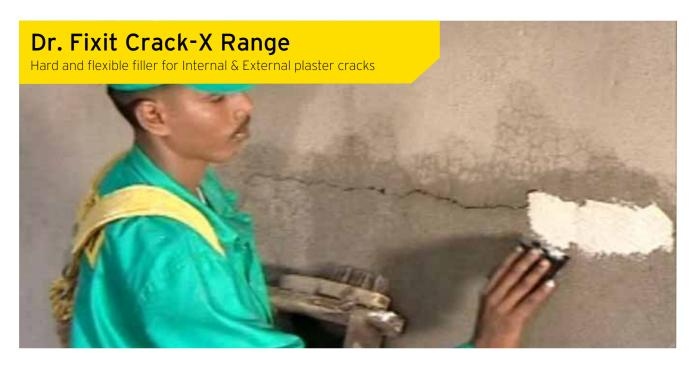
Ready to use crack filler for filling cracks on internal & external plastered brick masonry walls of up to 5 mm width
