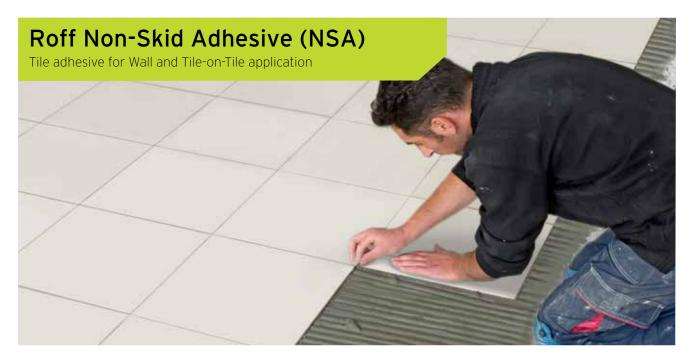
Ideal for tile-on-tile application. Fixing all kinds of tiles on floor & vitrified, large format ceramic tiles on walls.
