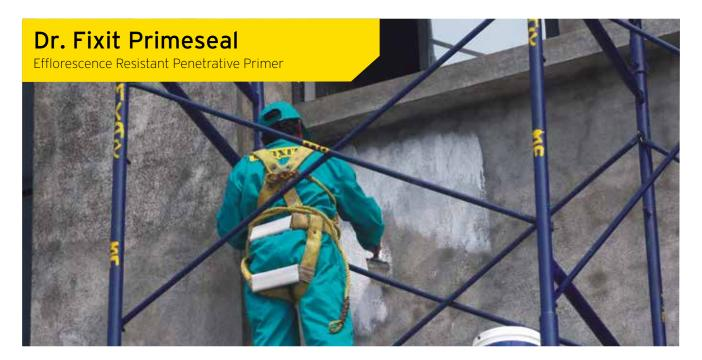
**Dr. Fixit Primeseal** is water-based primer composed of acrylic emulsion polymer, properly selected fine fillers, white pigments & additives in water as a medium. It is used as primer over exterior & interior building walls before application of water based paints.
