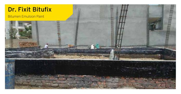
**Dr. Fixit Bitufix** is an emulsified thixotropic bitumen protective coating. The coating dries to form a black flexible protective film. The finished film forms a tough barrier to vapor transmission.
