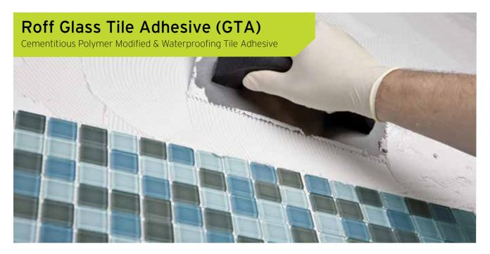
Fixing of marble slabs, glass mosaic, glass tiles on internal, external wall, floor surfaces & swimming pool.
