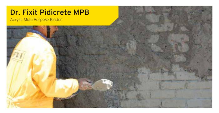
**Dr. Fixit Pidicrete MPB** is composed of acrylic co-polymer emulsions & additives. It is used as bonding agent for new to old substrates & cement mortar modifier because it provides strong bonds to old & new concrete. Improves tensile & flexural strength of concrete and increases the durability of the structure. When mixed with cement, It forms a matrix & provide excellent waterproof coating.
