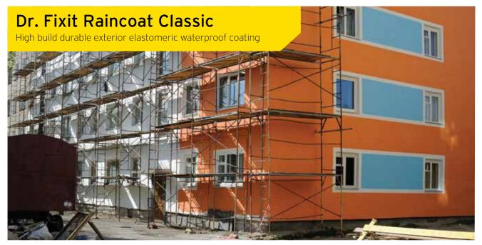
**Dr. Fixit Raincoat Classic** system is composed of high quality acrylic emulsion polymer, light fast & weather durable pigments, properly selected & graded fine fillers, additives & biocides. It is used as a waterproofing & protective coating for exterior walls of the buildings because it forms high film thickness. It has excellent flexibility, breathability, water resistance, crack-bridging, weathering durability and an excellent resistance to the growth of micro organisms.
